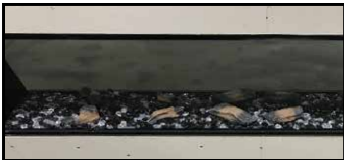
Figure 4.14 Media and Small Logs Installation
